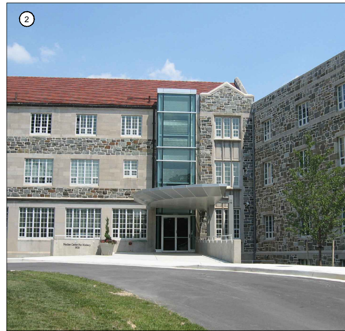
JUXTAPOSITION OF STONE WITH SMOOTH-SURFACE PANEL AND GLASS; COLOR AND TEXTURE SIMILAR TO EXISTING HECKER CENTER (ABOVE)
